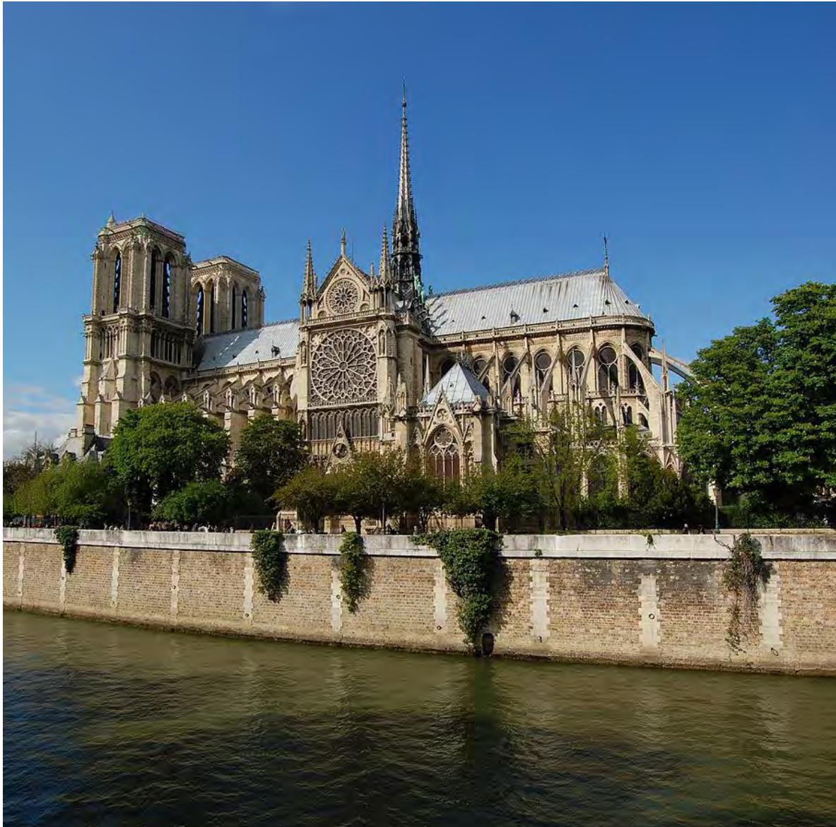
Figure 12 Notre Dame de Paris. It shows the characteristics of Gothic architecture born in the region of Ile de France in the late twelfth century: the use of the pointed arch and high vaults that shift the weight by way of the flying buttresses (clearly visible in the image), the predominance of the openings on the walls, which allow large rose windows, the height of the central needle and the central position of the transept. Wikimedia Commons Zuffe
